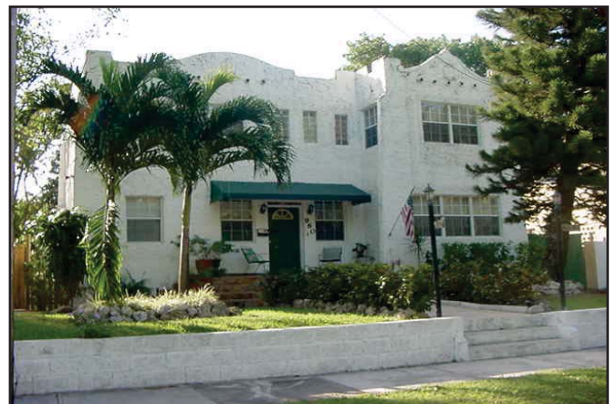
Two-story masonry house in Spring Garden
